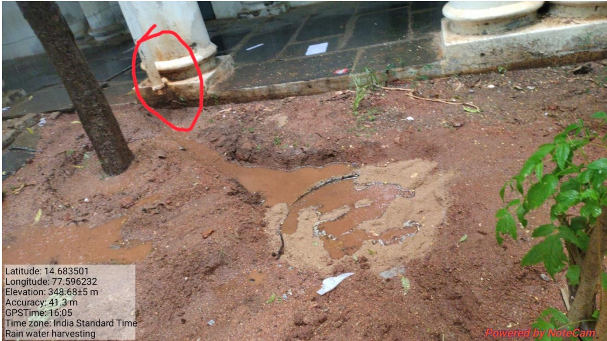
Water from the terrace drained to the percolation pits
