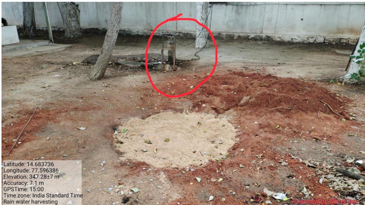
Recharge pit near the bore well
