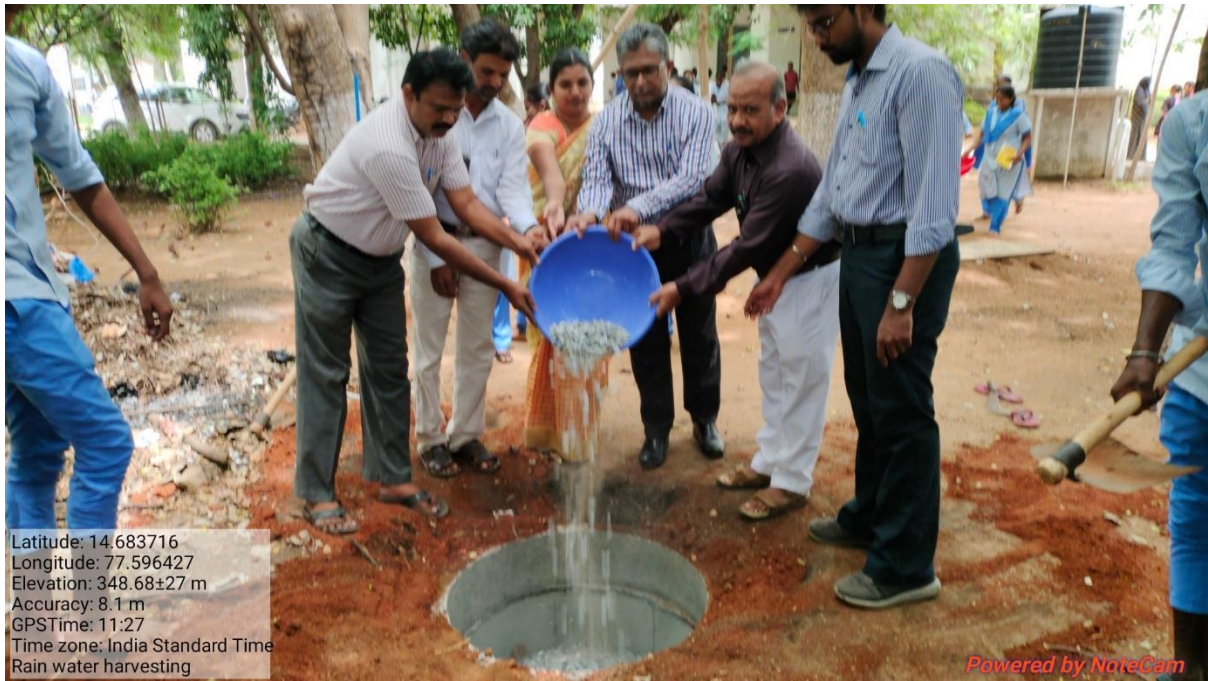
Filling the recharge pit with gravel and sand
