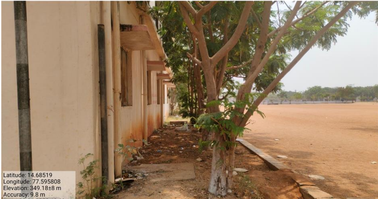
Luxuriant growth of plants with rain water from the terrace in the Commerce block
