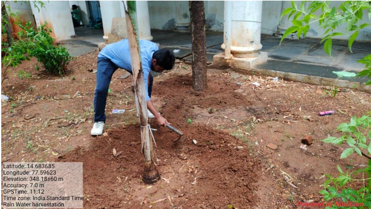
Channels made to drain water from the terrace water pipe.
